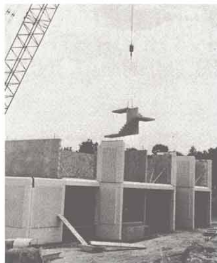
Stair tower interiors were fabricated in one-story sections and installed as a single unit.
