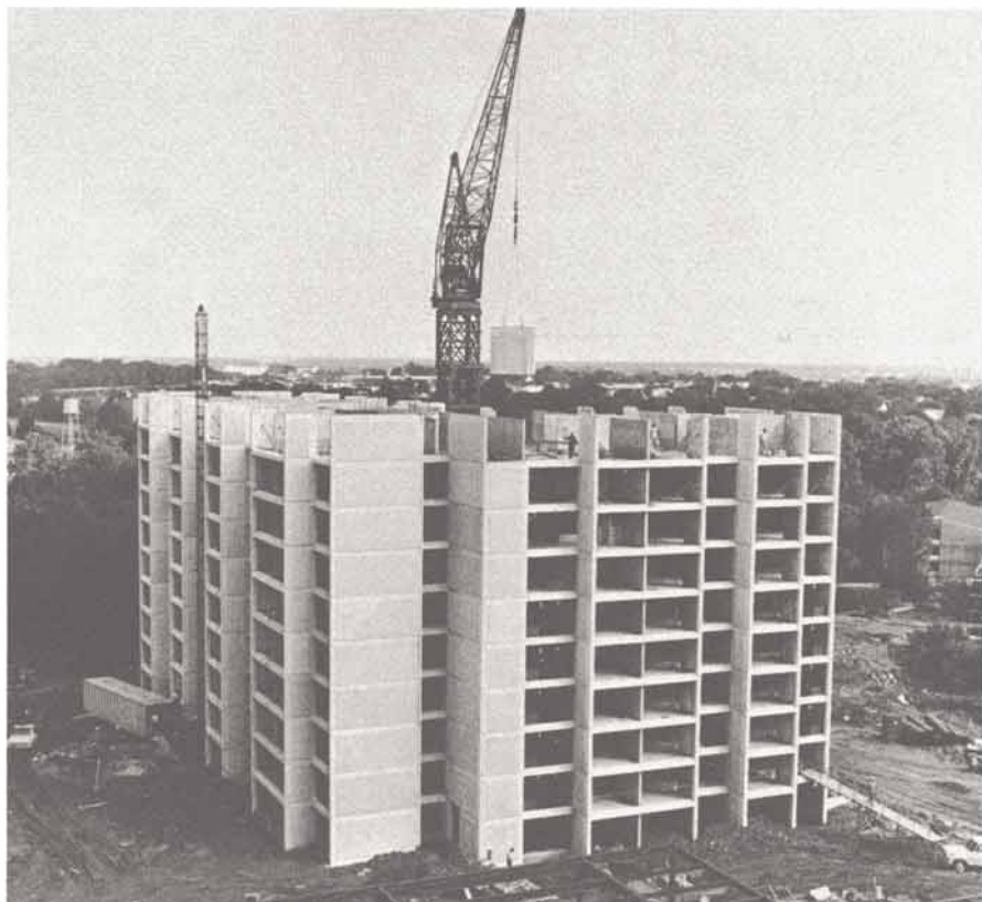
Exterior wall panel is lowered into place at one of student living towers.
