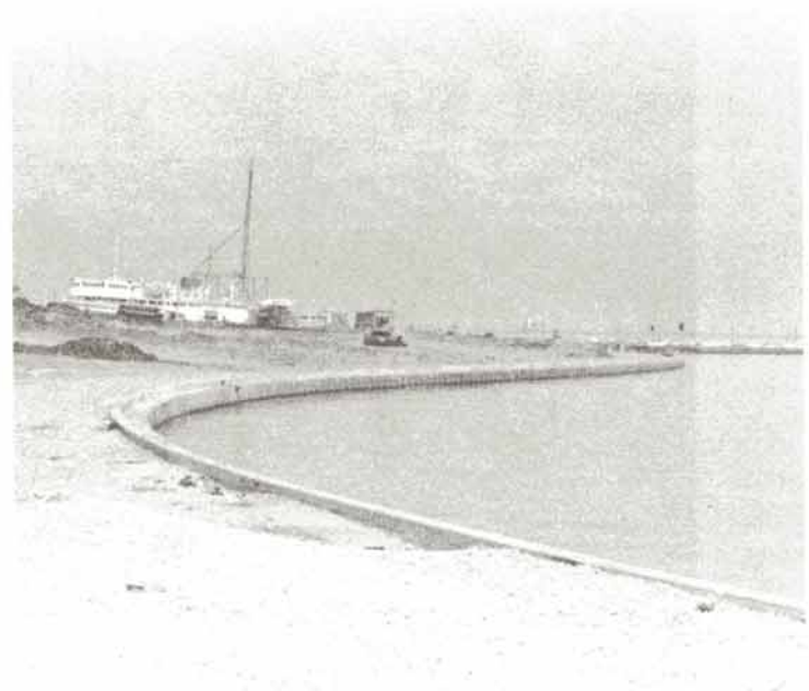
Photo 3 Bulkhead and Finished Backfill (Photo by Patrick Stack)
