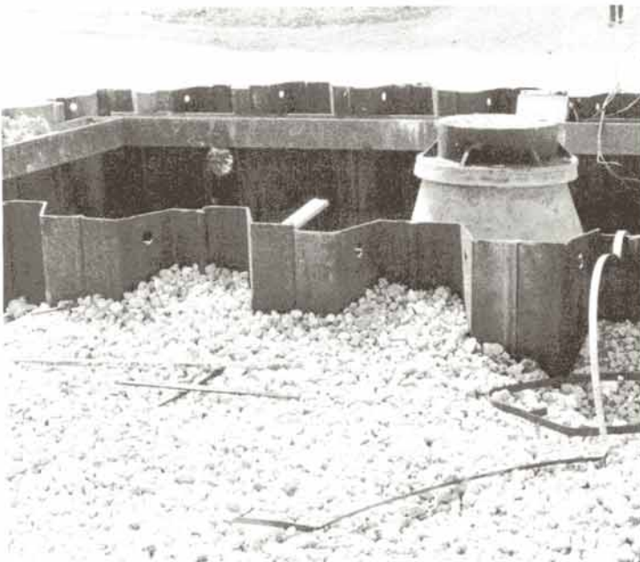
Photo 2 Typical Slag Fill Behind Bulkhead (Photo by Patrick Stack)
