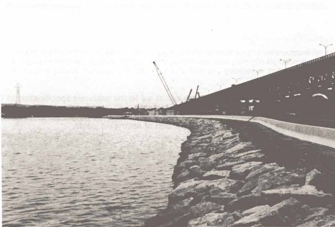
COMPLETED ROAD PROTECTED BY RIP RAP
