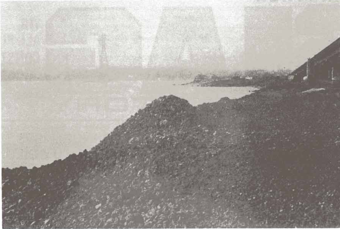
GENERAL VIEW OF BASE CONSTRUCTION
