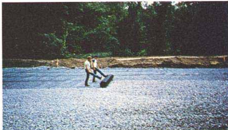
Geogrid material is unrolled on aggregate in preparation for next layer of aggregate.
