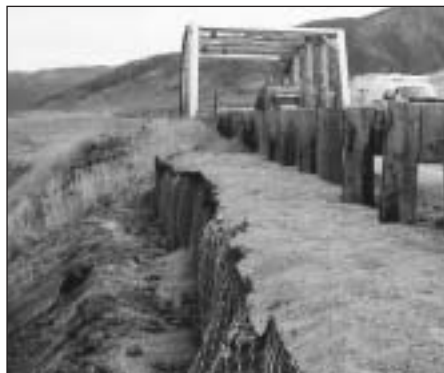
Slag-filled gabions.
