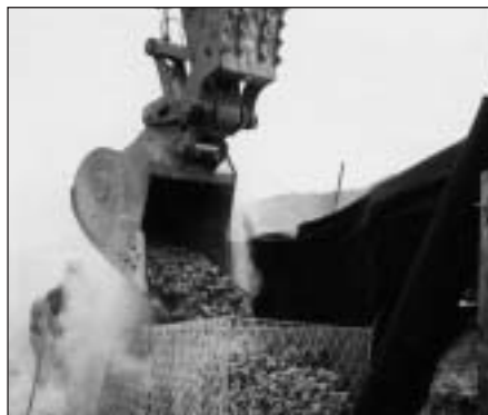
Filling the baskets with 2"-4" slag.
