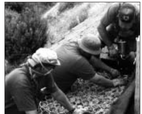
Road crew secures the gabion baskets.
