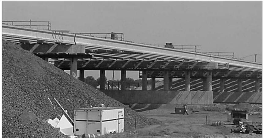
*Tons of ACBF slag help provide a cost-effective foundation as Michigan’s M-63 suspended roadway is replaced.*
