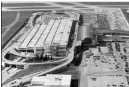
Construction nears completion, November 2001.
