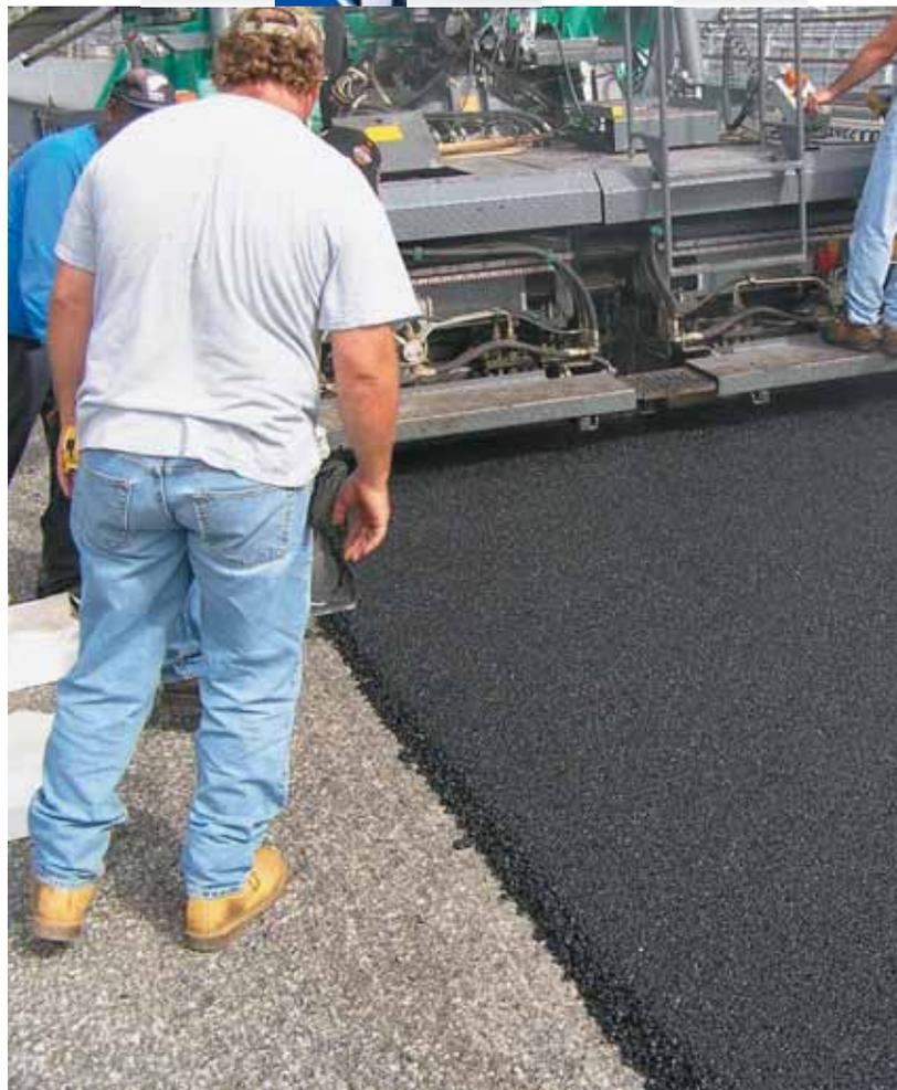
**Work crews laid the asphalt mat as close to the retaining wall as possible.**
