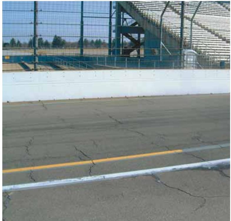
**The old track suffered from surface and reflective cracking.**
