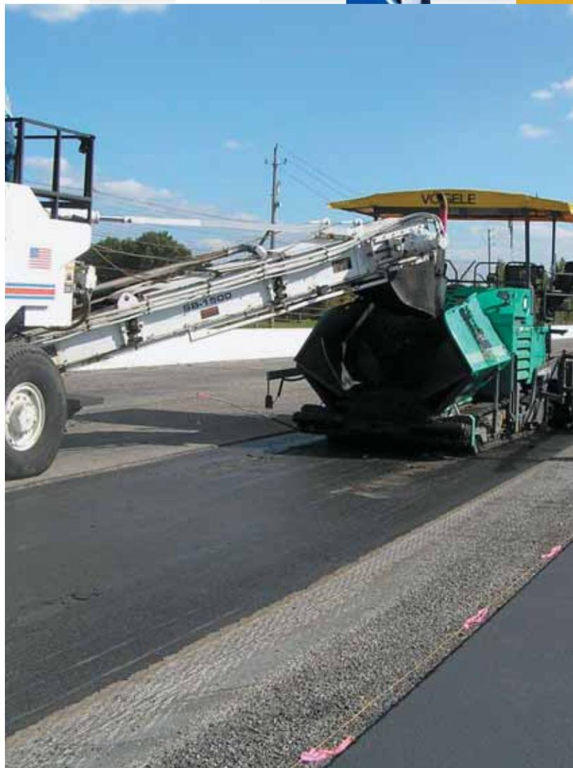
**The team from Grady Brothers used a consistent rolling pattern on a SMA mix to achieve at least 94 percent compaction. The crew used a consistent feed of material and a steady pace to complete one revolution of the 2.5-mile track each day. This procedure limited the number of joints in the mat.**
