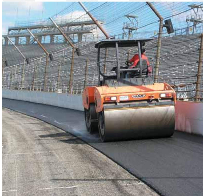
Roller operations had to be done with precision at the track.
