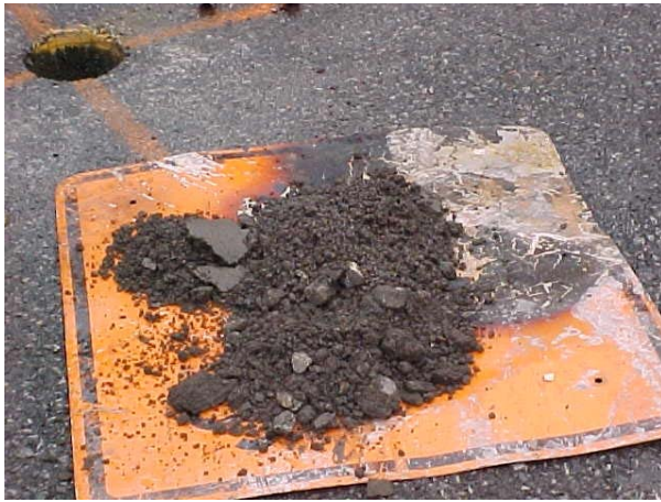
Figure 2 Core Made in Roadway
