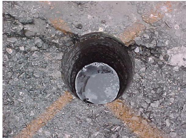
**Figure 3 Water Infiltration**
