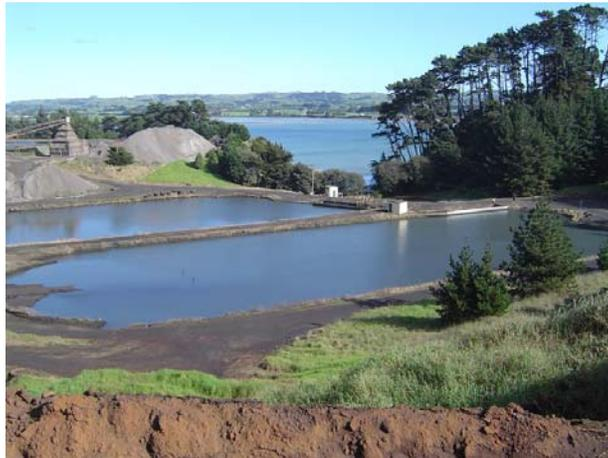
Figure 4 shows New Zealand Steel's main storm water settling ponds, which capture the solids from around the production units, roads, unsealed areas and SteelServ's stockpiles. Each pond size is 15,000m<sup>3</sup>.
