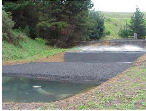
Water is sprayed across the top of the first bed, then drains through a second bed of coarser aggregate before discharge. The water volume is approximately 65m<sup>3</sup> an hour and the hydraulic residence time is only about two hours. Slag volume is just over 260m<sup>3</sup>.
