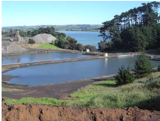
Figure 4: Northern side Storm water Ponds, NZ Steel
