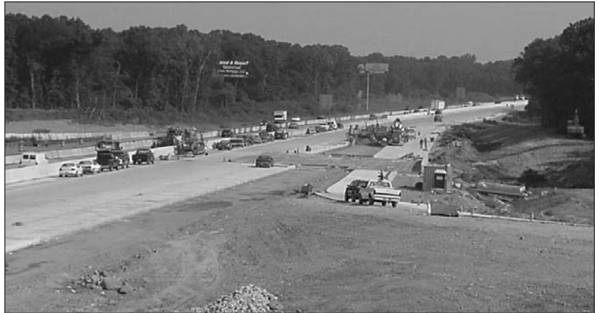
I-65 looking (north or south). Stage of completion?
