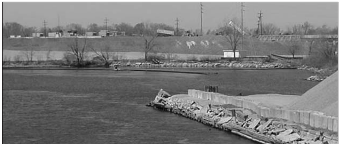
M-63 project, Benton Harbor, Michigan
