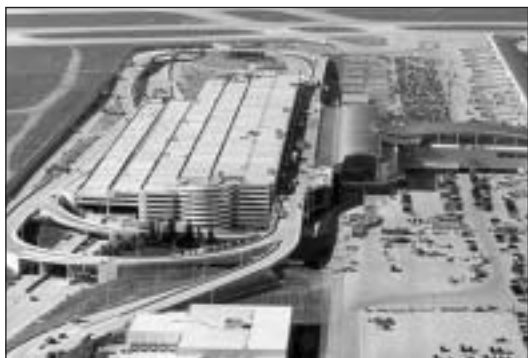
Construction nears completion, November 2001.
