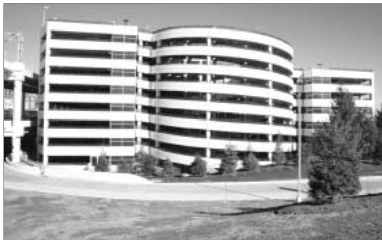
The completed parking garage structure at opening in February 2002.
