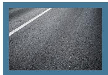
AN OUTSTANDING CHARACTERISTIC OF ACBFS IS ITS TOUGHNESS AND RESISTANCE TO POLISHING UNDER TRAFFIC.
